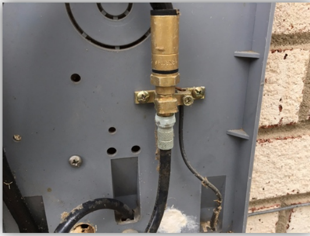
Figure 31: Twist on F-Connector at Ground Block
