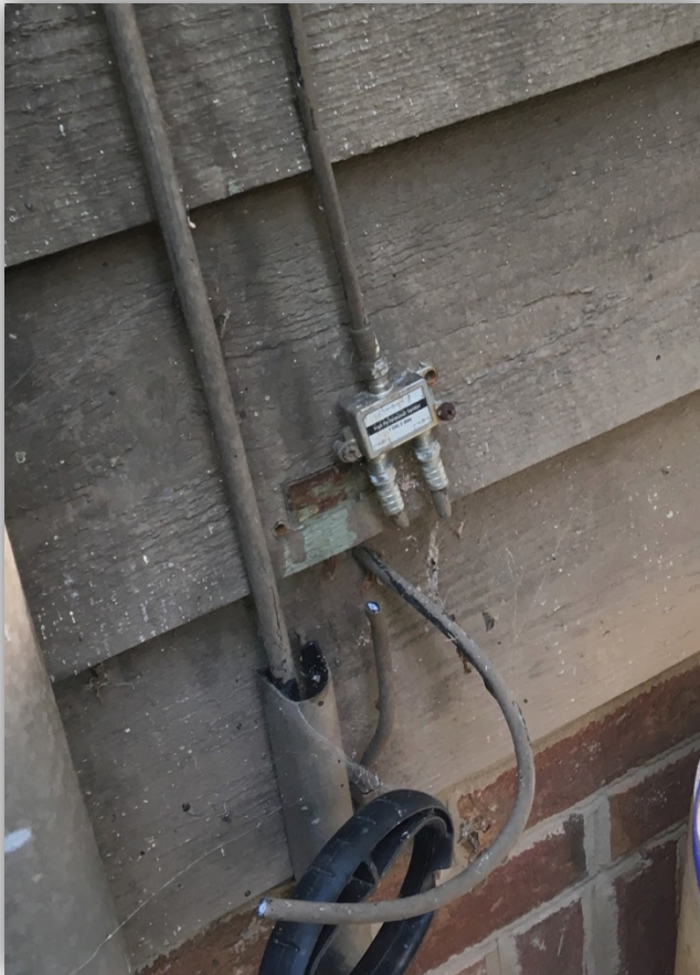
Figure 17: Old Splitter and Twist-on F-Connectors
