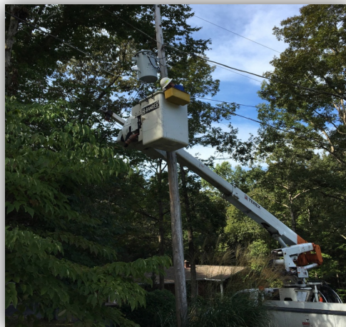
Figure 5: Technician installing M3 Signal Injector
