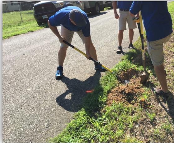
Figure 11: High Leak Location Being Excavated
