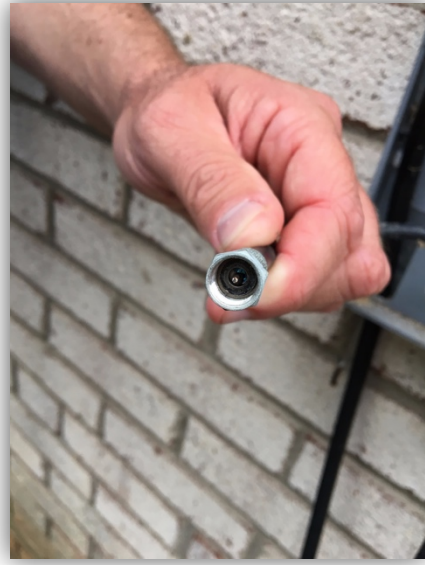
Figure 31: Twist on F-Connector at Ground Block
