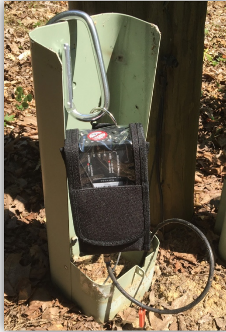
Figure 10: ComSonics' M3 Connected to Buried Subscriber Drop Cable
